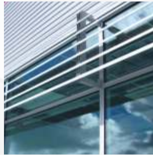
WINDOWS WITH IN BUILT AUTOMATIC LOUVERS
